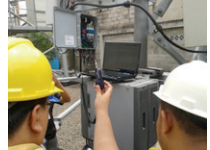
At the RRU (tower structure or rooftop)
